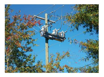
Devices using self-resetting interrupter technology can replace fuses on lateral lines. When a fault occurs, these technologies briefly interrupt power, then check to see if the fault has disappeared, automatically bringing the line
