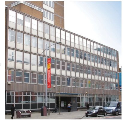
S&C's EMEA headquarters in Swansea, Wales.
